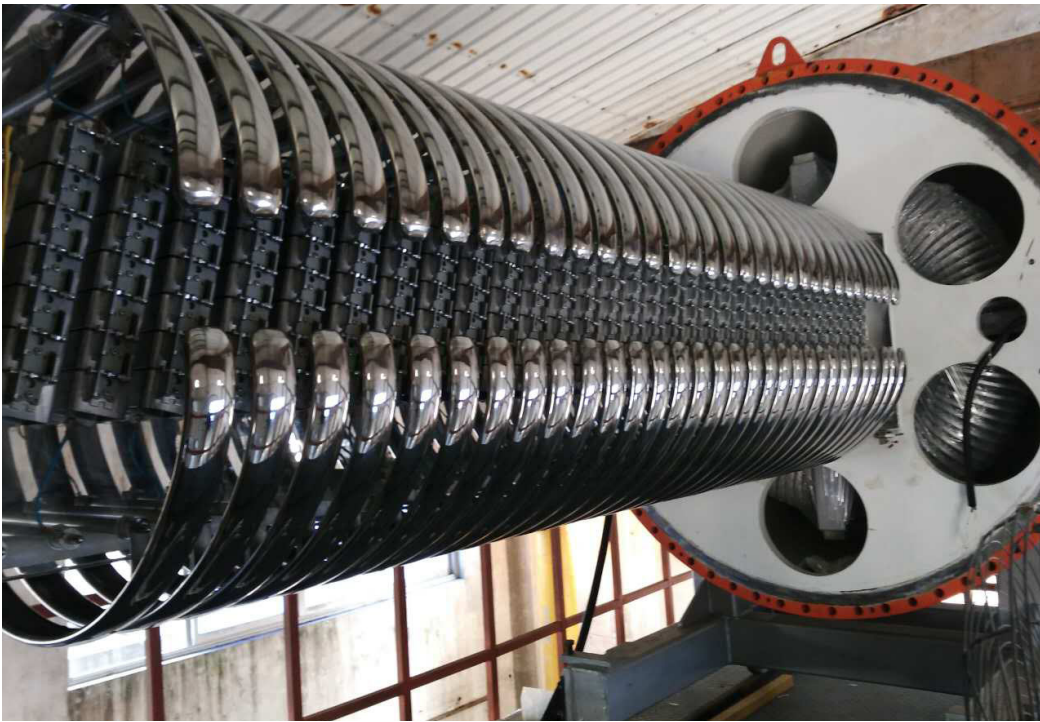
Electron beam technology is used to clean industrial wastewater at a textile dyeing facility in Jinhua city.
